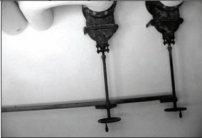
Fig. 62: Heavy insulated hot water (or steam?) pipes in the room behind the alleged gas chamber of Dachau camp, leading into the space above the current room. 1
