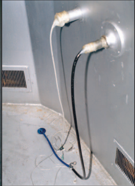
Fig. 108: Inside gas chamber where stethoscope and other body monitoring line enter. They are covered in Vaseline to indicate leaks. Fresh air vents on the walls close to the floor.
