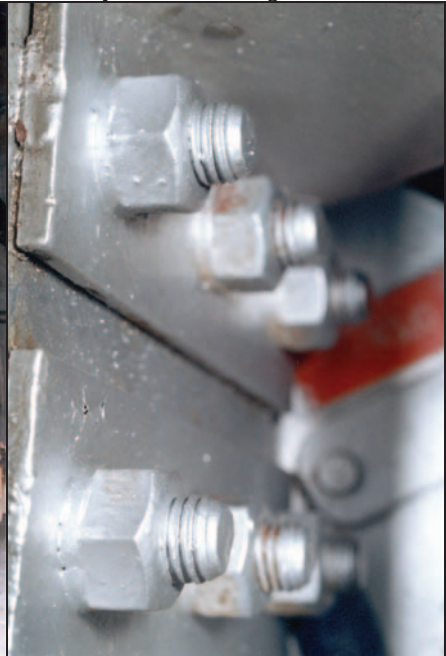
Fig. 106: Closeup of bolts on door hinges.
