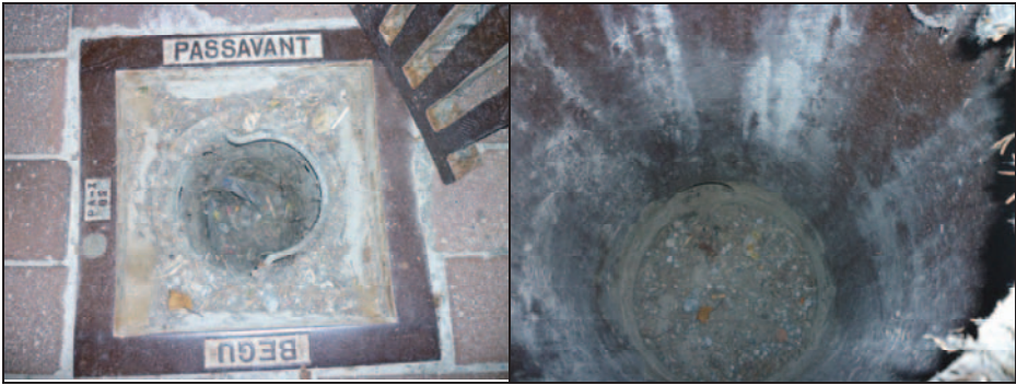
III. 60a & b: One of the six floor drains inside the alleged gas chamber at Dachau. Left: grate removed, sieve in place; right: sieve removed; the exit drain pipe can be seen at the drain's bottom (top-most spot of the bottom).
