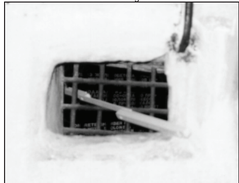
Fig. 33: Opening with grate in the wall of Room I in the disinfection wing of Building 41, Majdanek (see Fig. 31)
