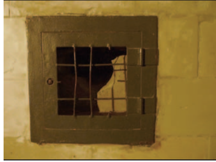
Ill. 58: Peephole viewed from within the chamber.
